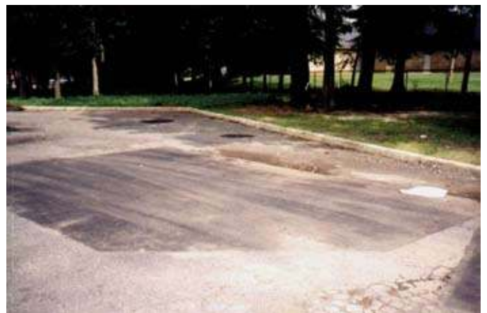
After INFRARED Restoration
