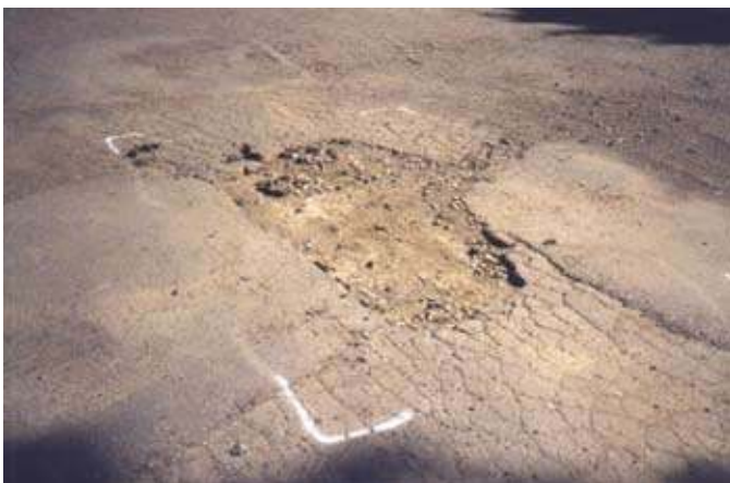
Alligator cracked area (before)
