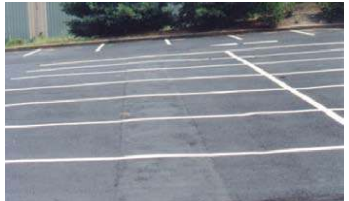
After INFRARED Restoration
